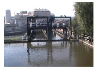
The lift consists of 2 caissons (tanks) which could be 'sealed' at either end and would hold 2 boats at a time. The caissons were raised and lowered on hydraulic rams between the two waterways where the appropriate end could be opened and the boats depart / enter. Problems were encountered over the years and a serious accident closed the lift for 6 months in 1882, the same year that grooves were first noticed on the hydraulic rams.
